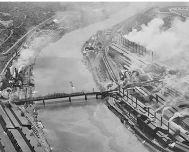
Jones and Laughlin steel mills on each side of the Monongahela River c1951. The shore on the left is now a technology park, while the right shore is now the home of the South Side Works. Source: Carnegie Library of Pittsburgh
